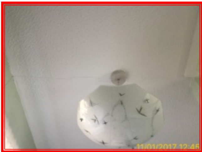
6.1.1 Please see wall description.
